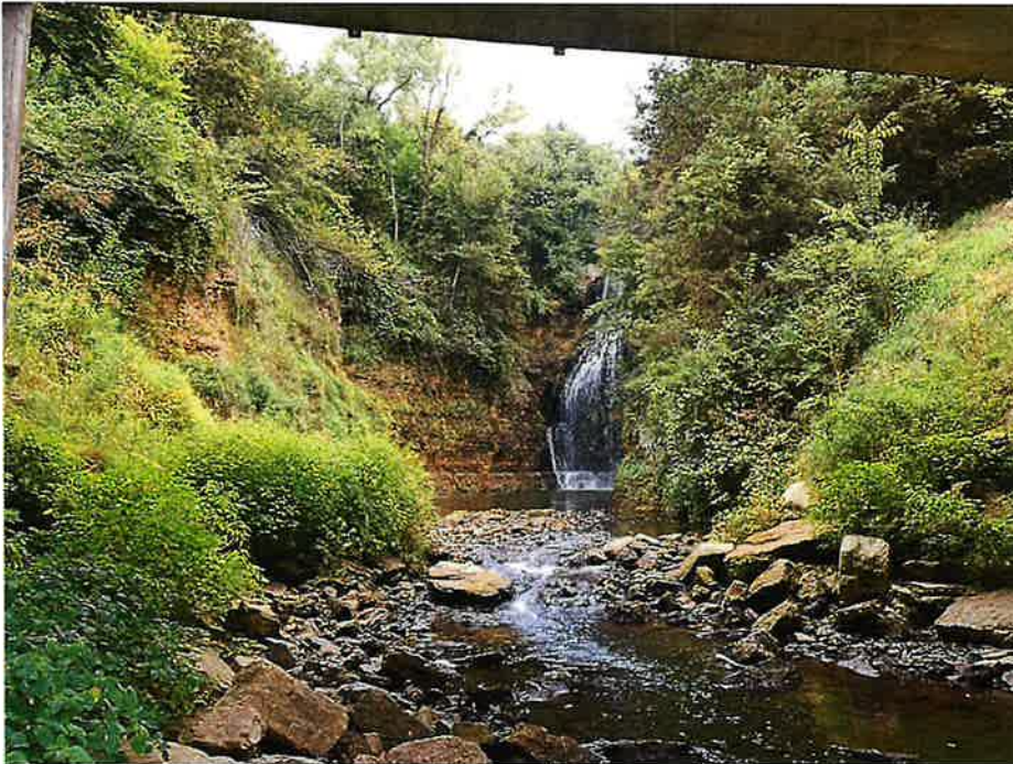
View upstream of bridge on South Apple Canyon Lake Road
