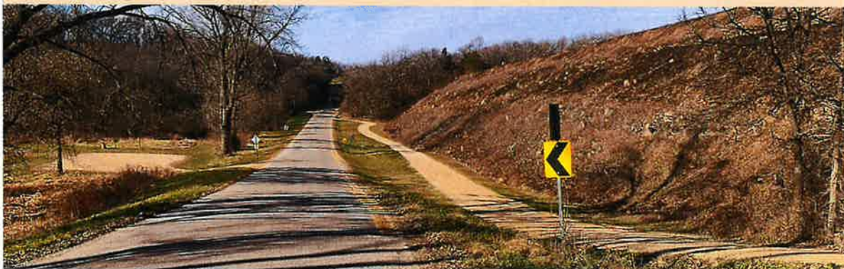
Photo: Downstream Face of Dam looking NW
