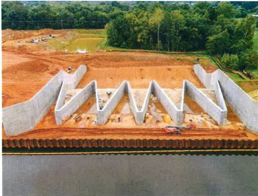
Figure 1 – Labyrinth Spillway Examples
