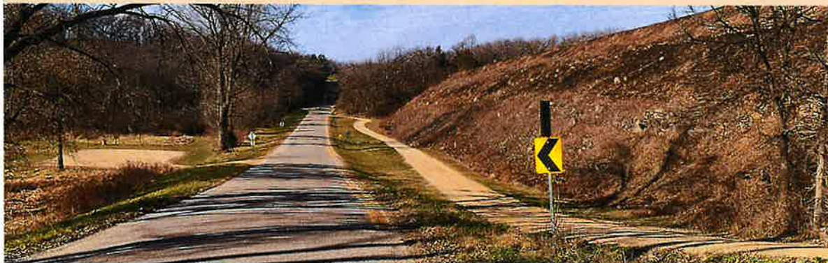
Photo: Downstream Face of Dam looking NW
