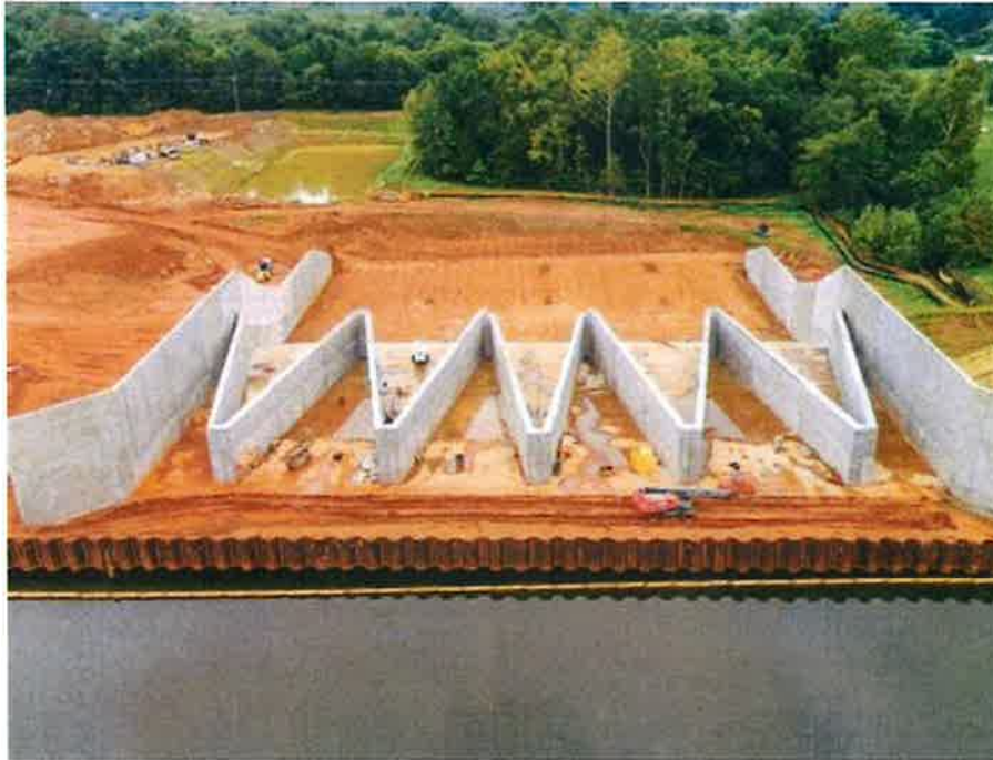
Figure 1 – Labyrinth Spillway Examples
