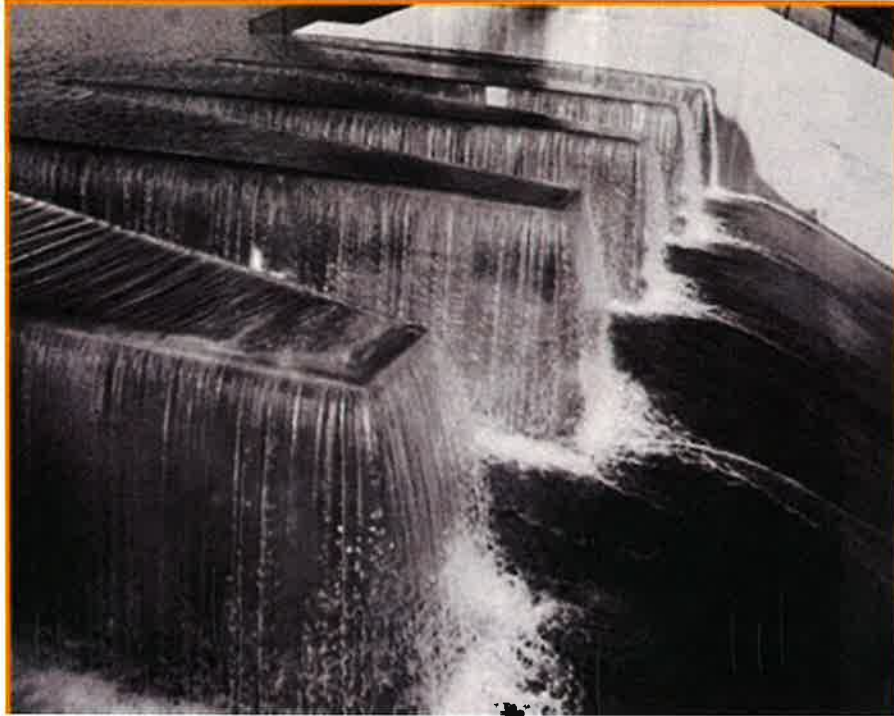
Figure 2 – Labyrinth Spillway Example
